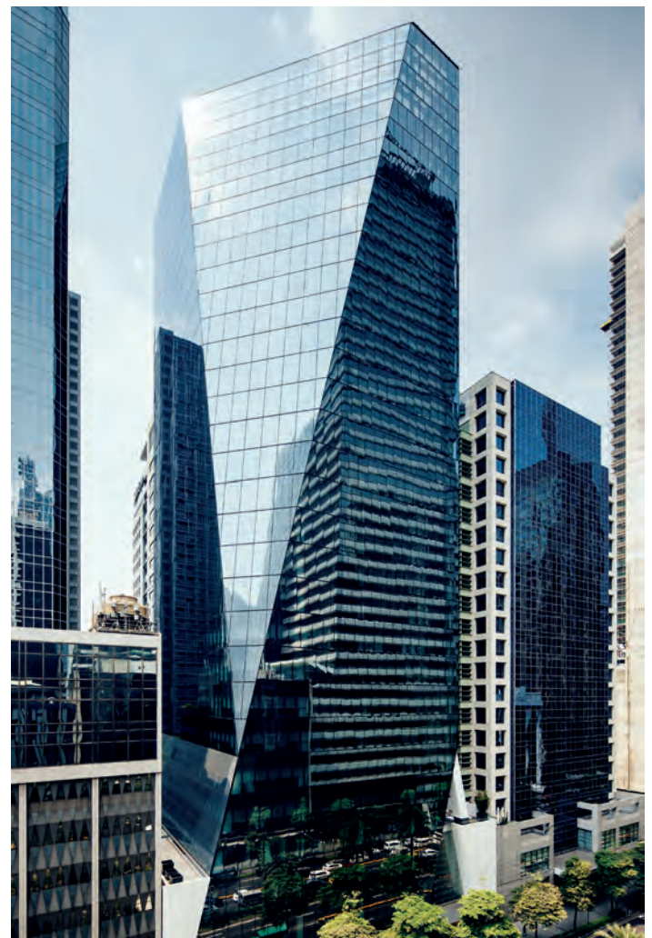
Nex Tower features a simple crystalline geometry. Photo: © Studio Periphery
